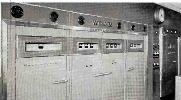
WQAM—MIAMI —The clear, strong signal from this station blankets greater Miami and gives dependable coverage of the 15 additional counties in its trading area. Above: G-E 5 kw AM transmitter. (left), Monitor rack, G-E 10 kw FM transmitter (background).
